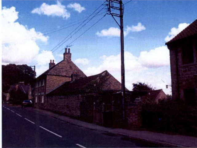
Fig. 3: View of site from north west, showing west wing in foreground
