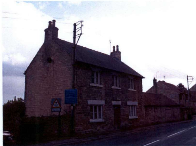
Fig. 2: View of site from north east, showing house in foreground
