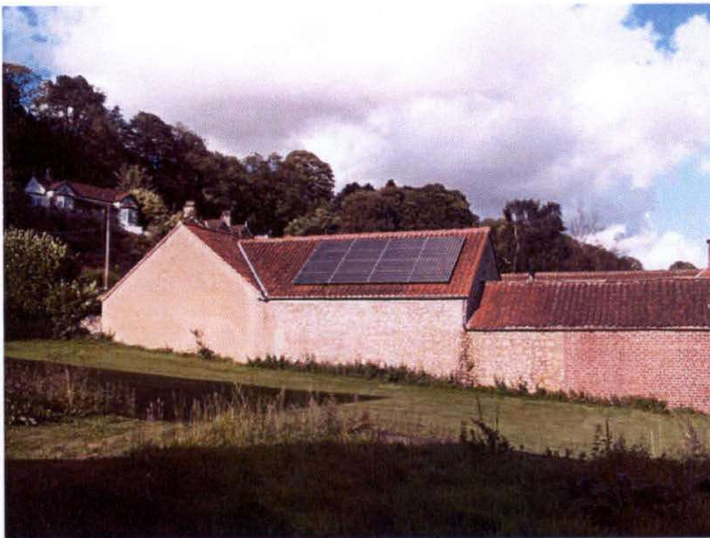
Fig. 7: Developed out-buildings to The Red House on eastern boundary
